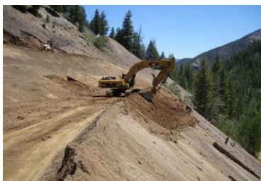
Ramshorn Mine Remediation, Bayhorse, Idaho
